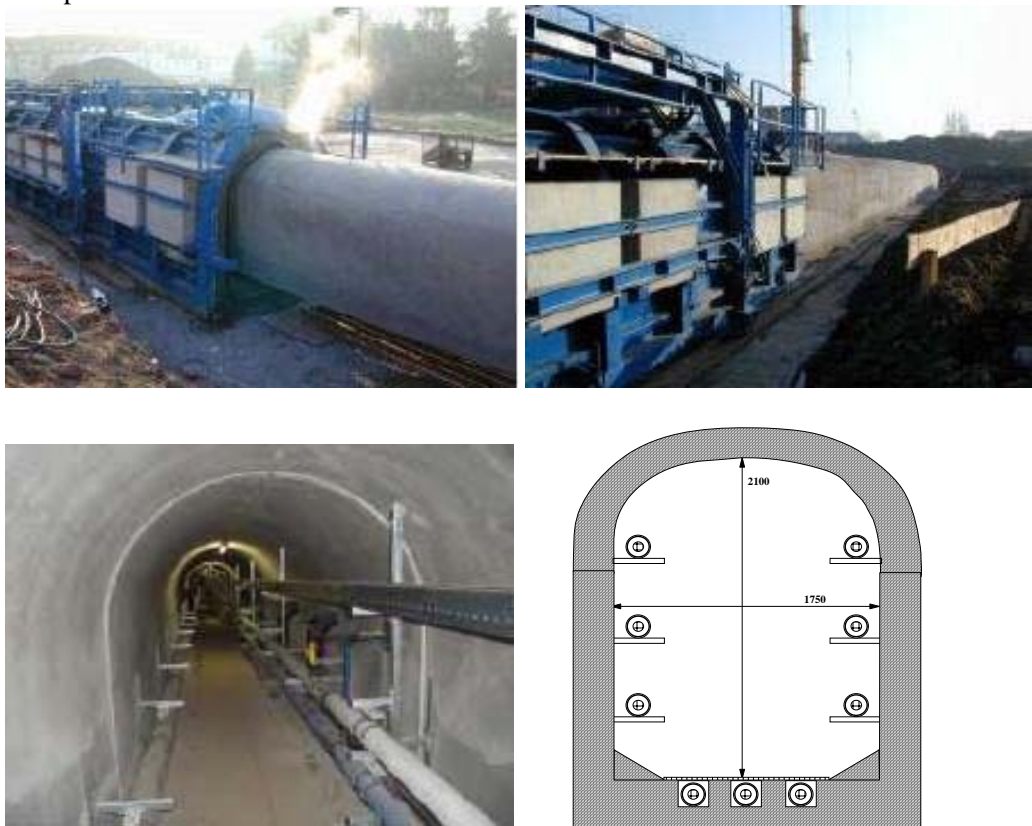
Figure 75 Infrastructure tunnel, system Dupré, Speyer; above: construction works, below left: installation of equipment in the tunnel, below right: schematic drawing of tunnel cross section with three UGC circuits
